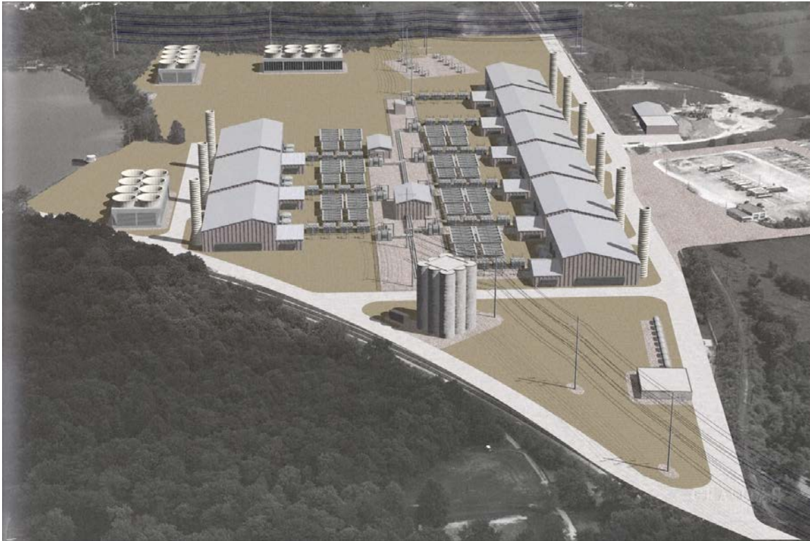
Figure 9: A rendering of the proposed 2700 MW CAES plant based on an abandoned limestone mine in Norton, OH
