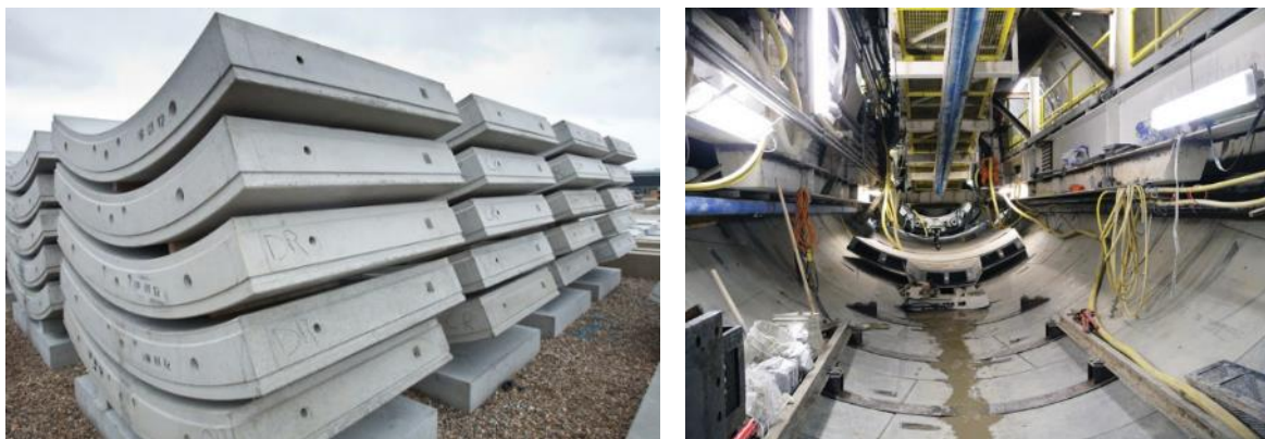
Figure 20: Examples of precast segments for tunnelling applications
